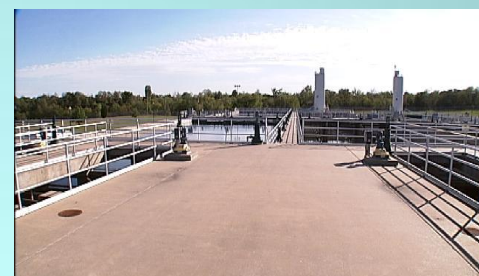
Mohawk Water Treatment Facility, Baucum
